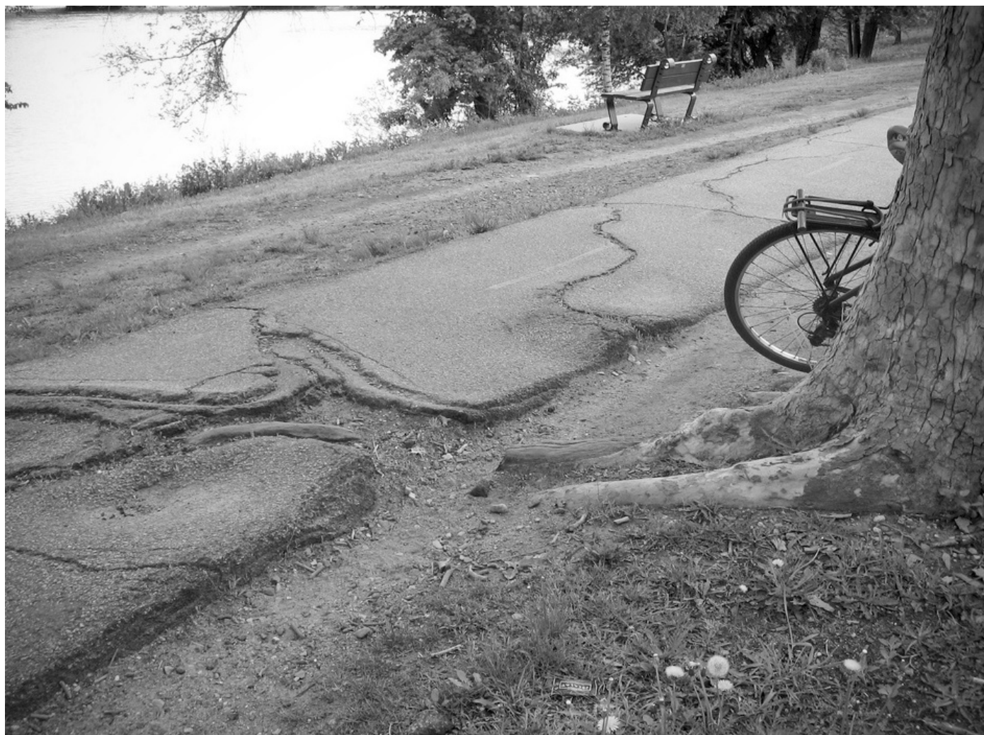
Where sidewalks are properly designed using specifications appropriate to the soil type, they are more able to resist being moved by growing trees. Of course, matching trees, based on size at maturity, with available growing space is important, too.
