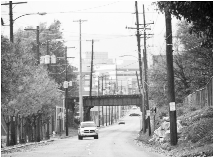
If extra tall poles can be used to span overpasses, they also offer potential for use around tall trees.
